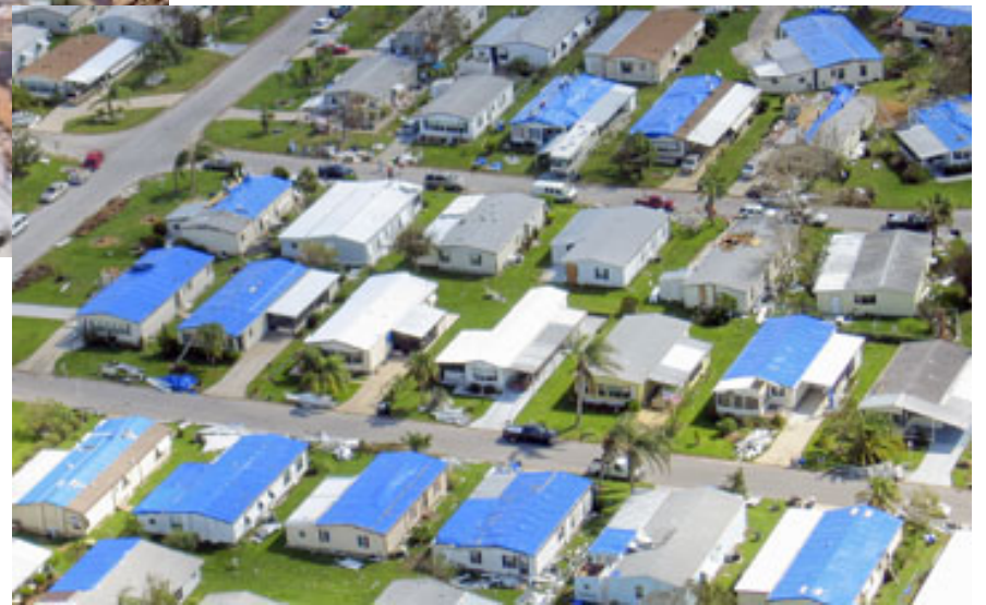
Houses with damaged or missing roof sheathing in Florida
