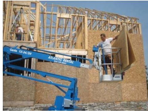
Mechanical Lift to Bring Plywood to Roof
