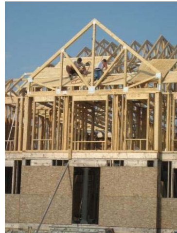
Application of Roof Sheathing Panels
