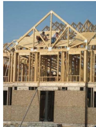
Application of Roof Sheathing Panels – New Construction
