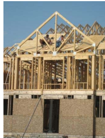
Application of Roof Sheathing Panels
