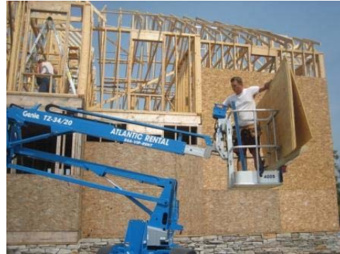
Mechanical Lift to Bring Plywood to Roof
