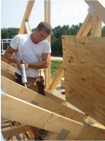
Adhesive Application to Roof Truss Top Chord
