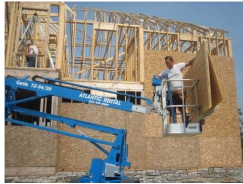
Figure 3 – Lifting Panels up to Roof Line
