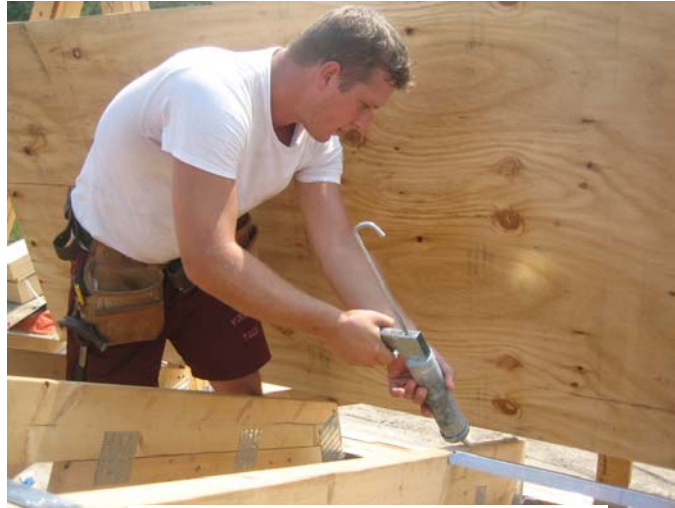
Figure 6 – Applying Adhesive
