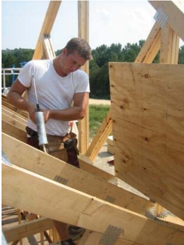
Figure 5 – Applying Adhesive
