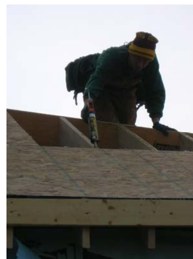
Picture 7: Applying the adhesive while the sheathing panel is being cut.
