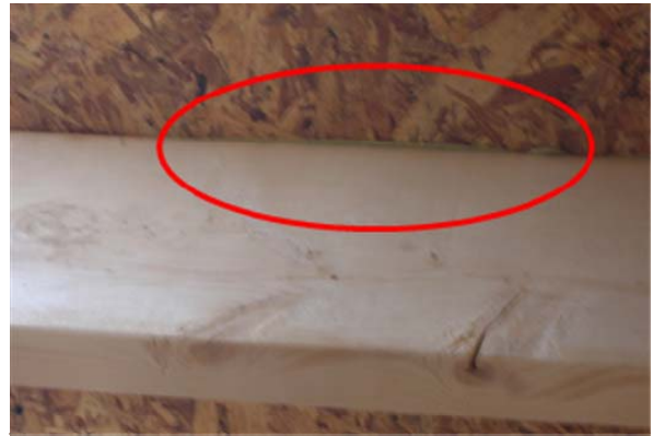
Picture 10: Adhesive pushed to edge of framing member.
