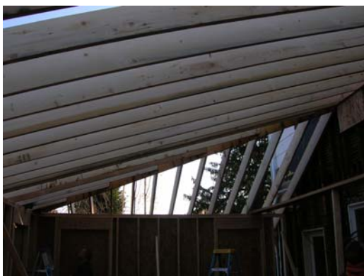
Picture 2: A picture from inside the addition.
