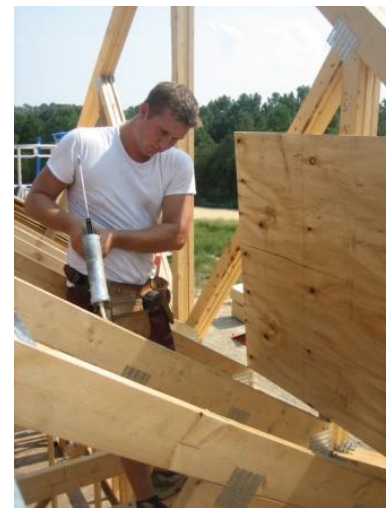
Picture 6: Applying the adhesive, with sheathing panel waiting in place.
