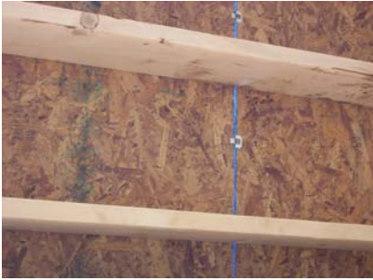
Picture 8: H-Clip on roof sheathing.
