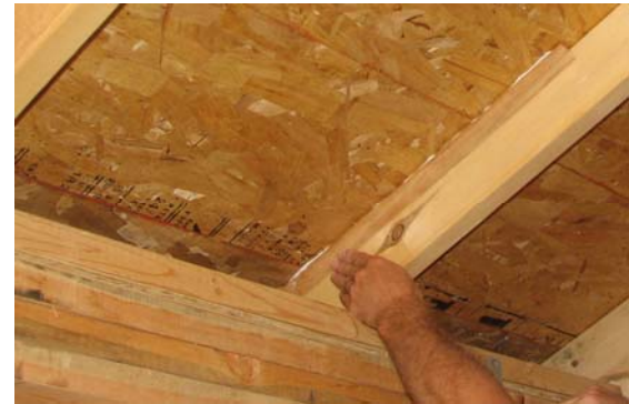
Placing quarter round into eave using the quarter round technique.
