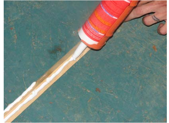
Pre-applying adhesive to quarter round on attic floor.
