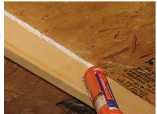
Applying adhesive on truss-sheathing connection using a standard caulk gun.
